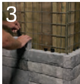
3 Attach Tandem Veneer with Connector
